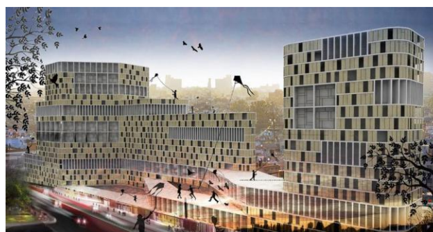
Fig No.5.2.2 Figure showing Mazgaon Chawl After Redevelopment
