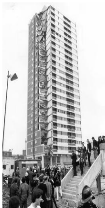
Fig.1. Ronan point after collapse.
